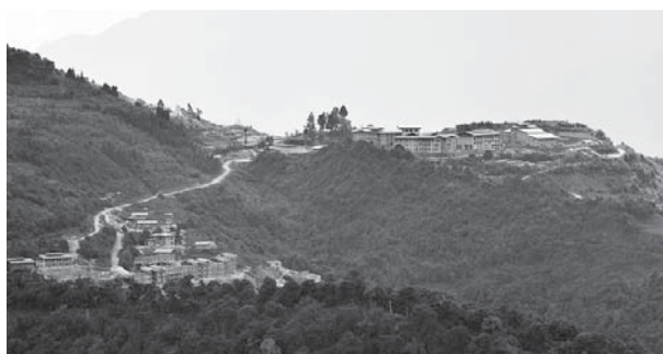
The new ILCS campus in Taktse, Trongsa
